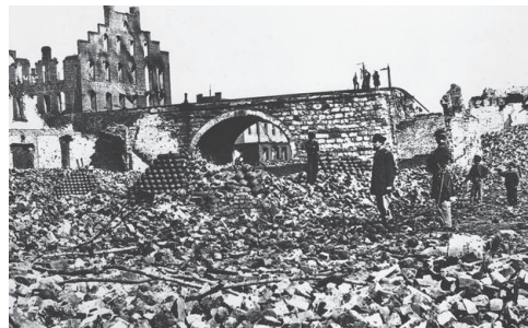
Matthew Brady, Ruins of Railroad Bridge, 1862
